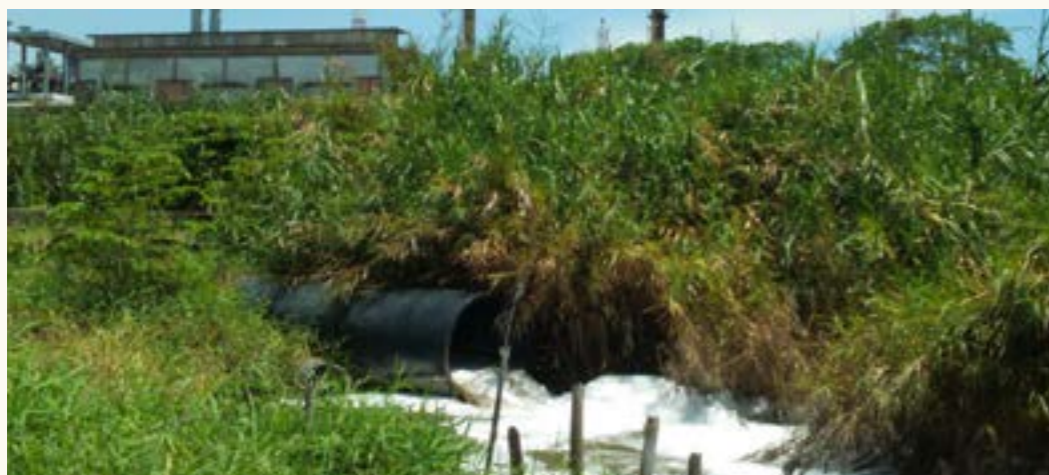
Discharge pipe with IBR factory in the background owned by Aditya Birla.
